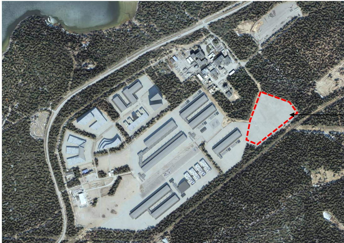
Future solar power plant
